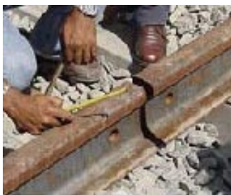
Fig. 3.2: Adjusting the initial gap
