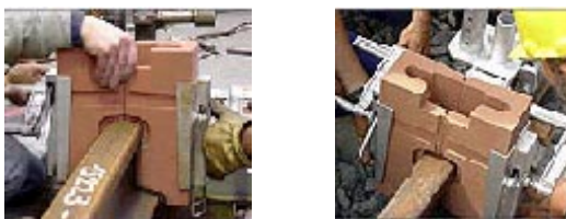
Fig. 3.4: Fixing of moulds and mould shoes
