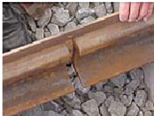
Fig. 3.3: Alignment of the rails
