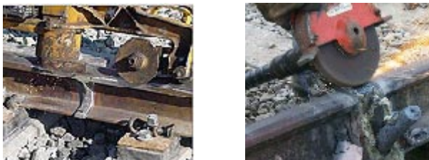
Fig. 3.9: Grinding operation
