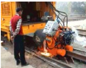
Fig. 2 : Flash butt welding by mobile unit
