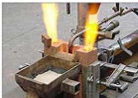
Fig. 3.6: Pre-heating of the rail ends
