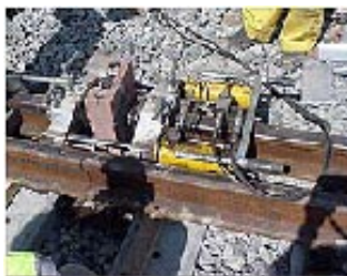
Fig. 3.7: Trimming operation by hydraulic weld trimmer
