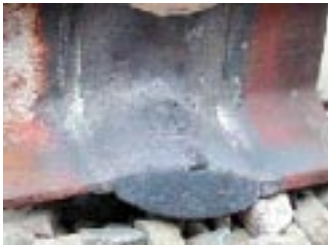
Fig. 3.12: Combination joint
