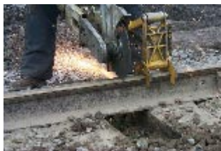
Fig. 3.1: Abrasive disc cutter
